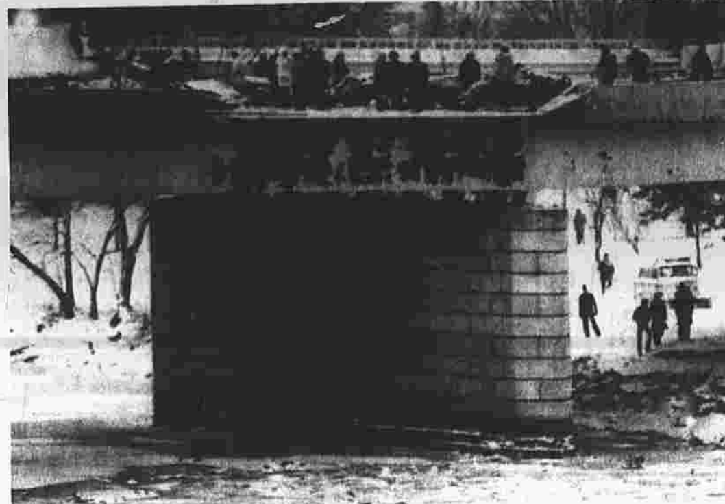
Rescue workers go over the wreckage of the 14th Street Bridge where the Air Florida jet crashed Wednesday, shearing off the tops of at least five vehicles.
